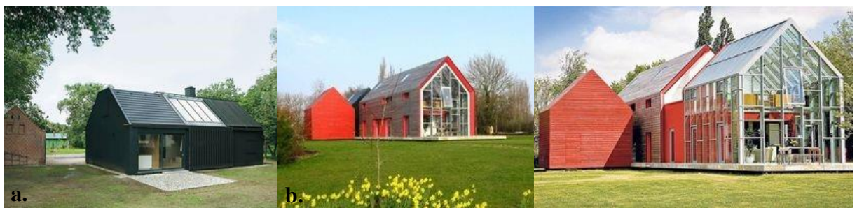
Figure 44: a. House in Oderbruch, Allemande, b. Sliding House Suffolk, Reaume-Uni, source : https://www.pinterest.ca , consulté le: 03/05/2021
