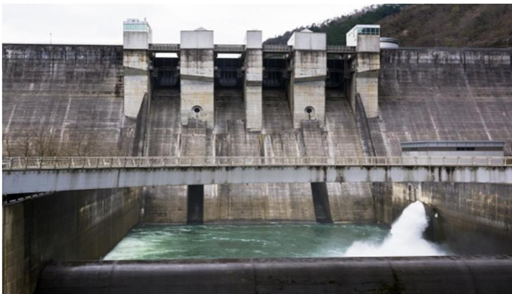
*Figure I.4: Barrage-poids. [3]*
