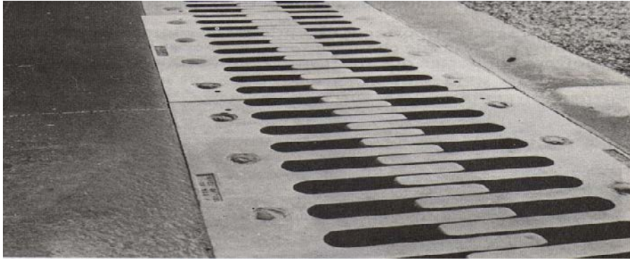
Figure 11.5: joint de chaussée (type WP alu.300)
