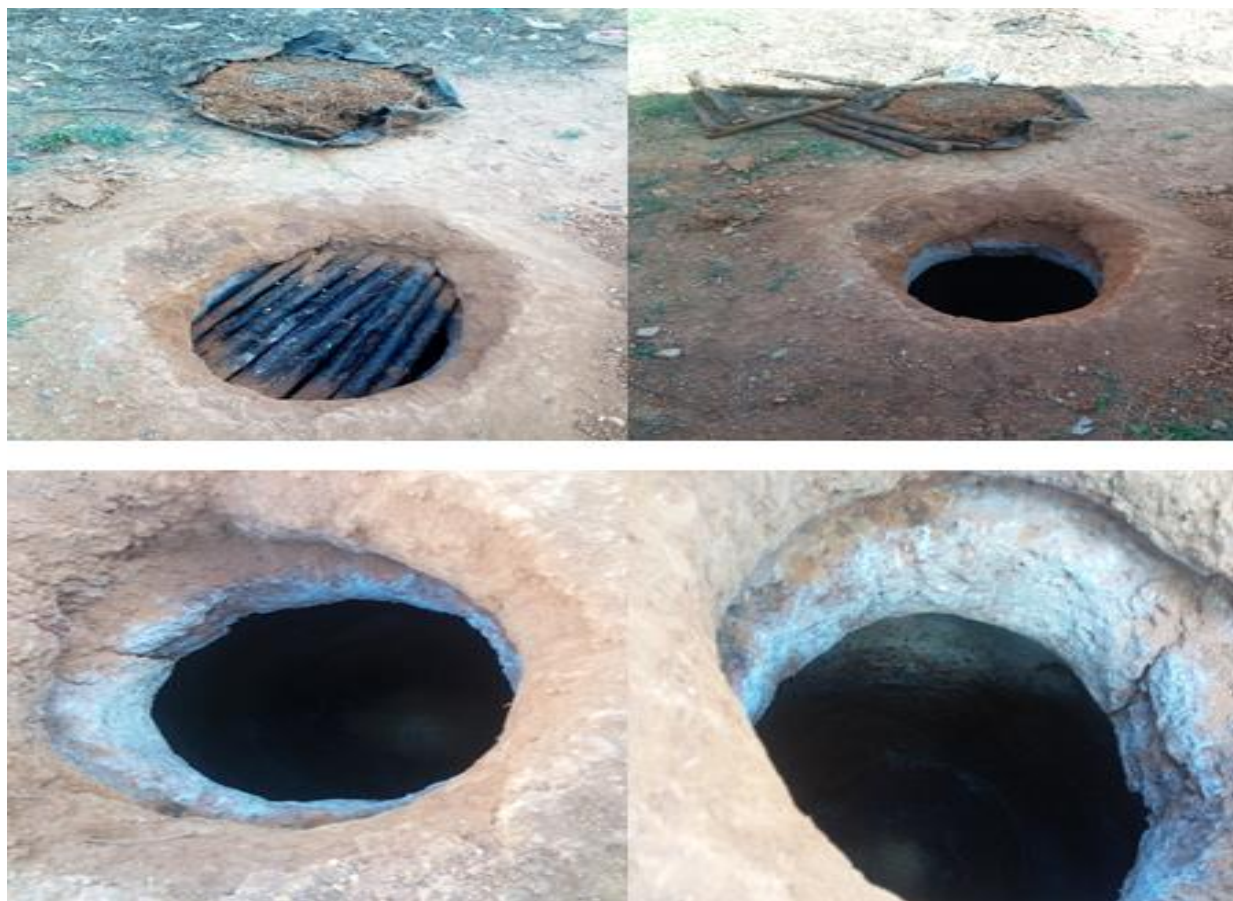
Fig. 7. Appearance of a ‘Matmour’ ( original photos ). This ‘matmour’ represents one of the fermented wheat sample collection sites, located in the commune of Boudria BeniYadjis, Wilaya of Jijel, Algeria. This underground silo can expand to about 5000 kg.
