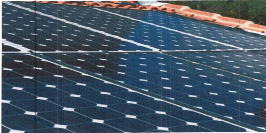
Figure I.5: Cellule en silicium monocristallin.
