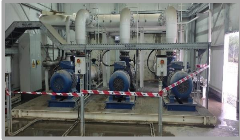
Figure 1.10 Transfer pumps
