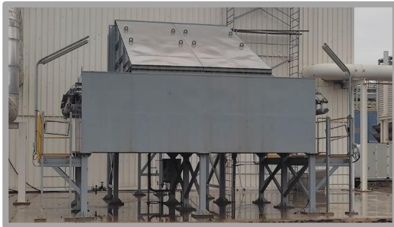
Figure 1.1 Air inlet filter
