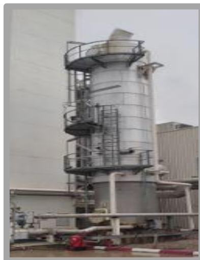
Figure 1.4 evaporation cooler
