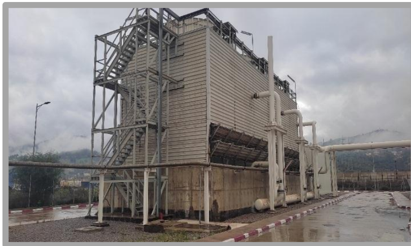
Figure 1.11 Cooling tower
