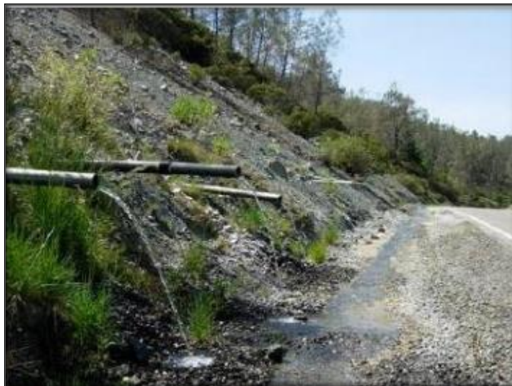
Figure II.01: Drainage de talus.
