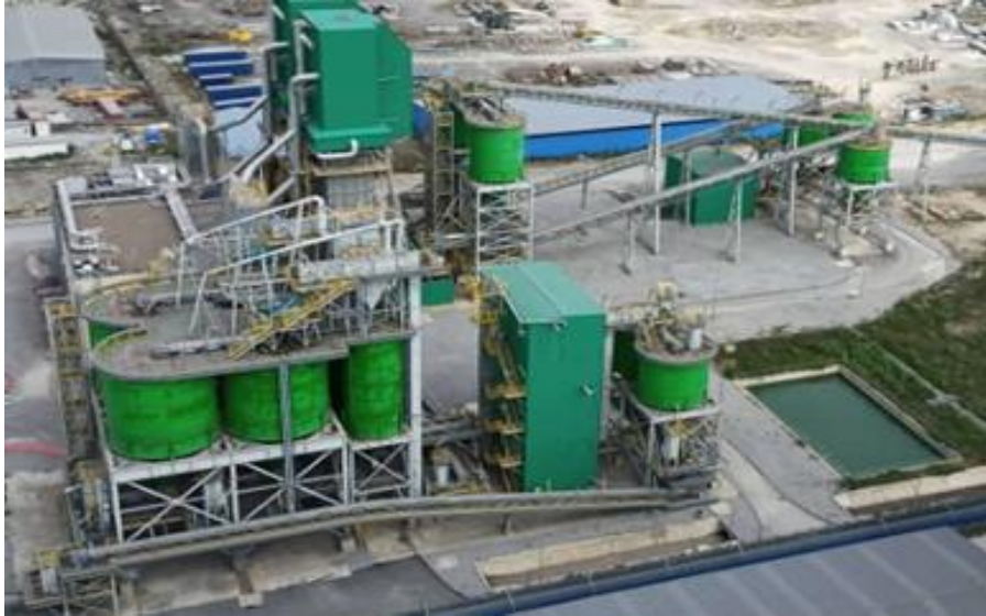
Figure I.4. Lime production unit.
