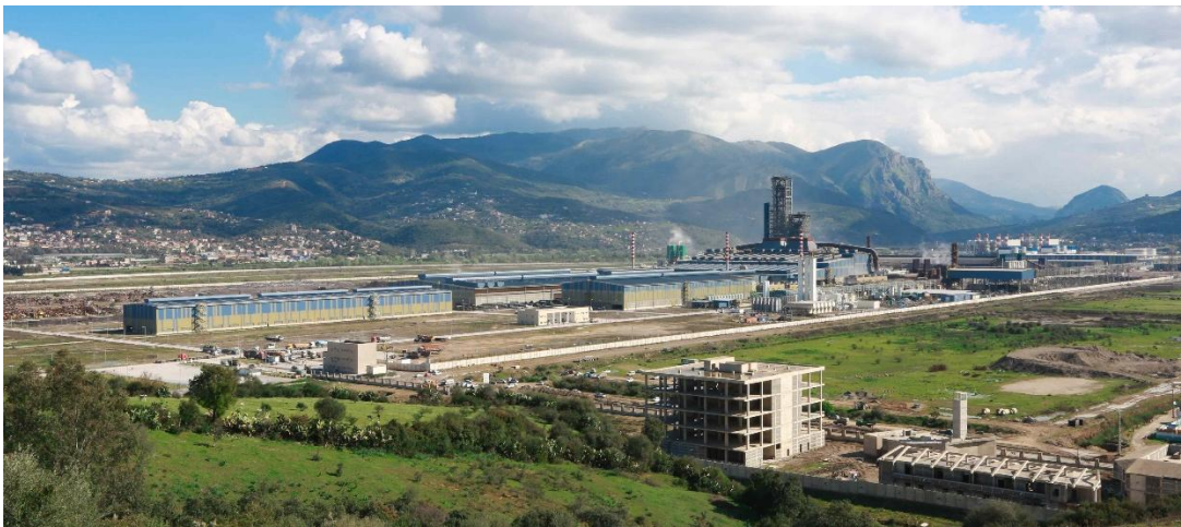
Figure I.1. Aerial view of AQS steel complex.
