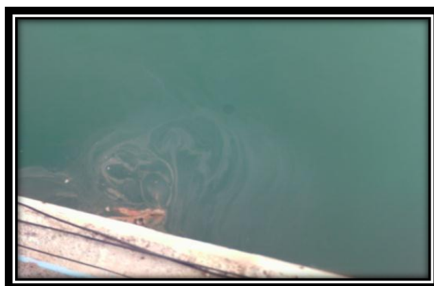
Photo 5. Station de pompage
