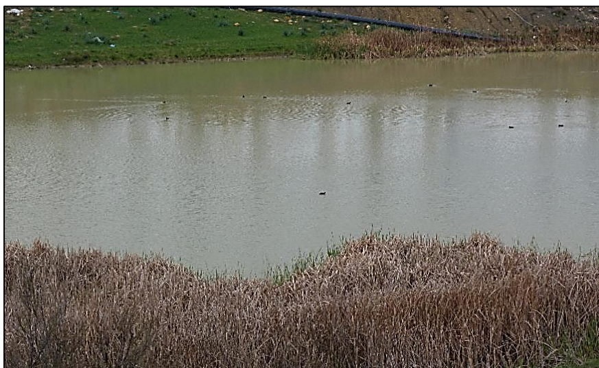
Figure 5 : Retenue collinaire Kharrouba (Original, 2018).
