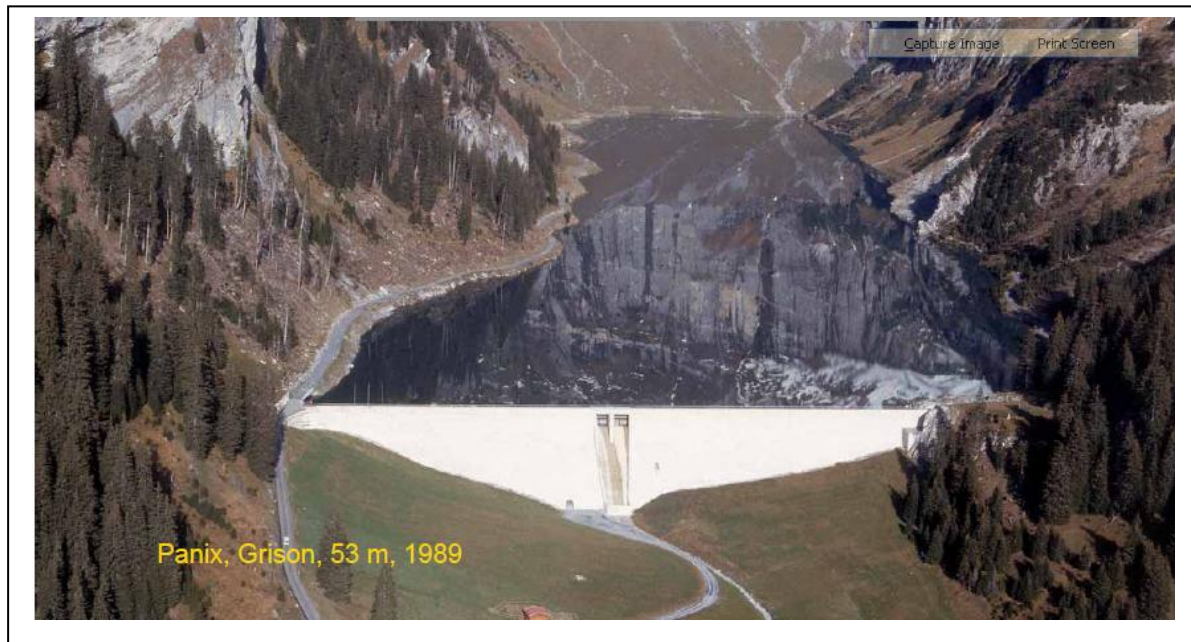
Figure I-3 :Barrage poids (Panix, Grison-1989).
