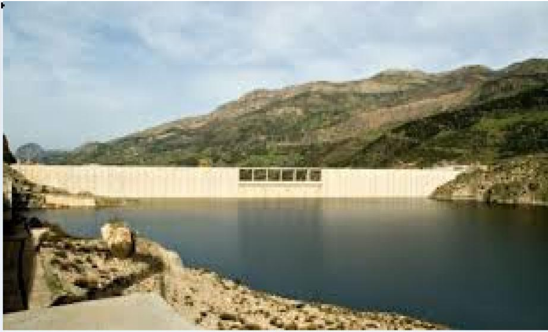
Figure II .1: Barrage de Cheffia.
