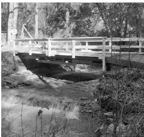
(Stream and bridge.tiff)
