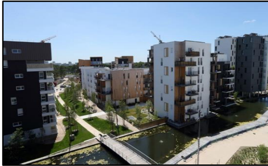
Figure 3-13 : ginko écoquartier (Source: https://un-balcon-s-effondre-dans-un-Eco- )
