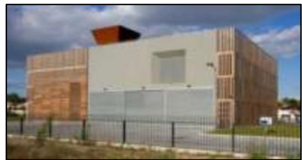
Figure 3-15 : Chaufferie biomasse (Source : Richard Bonnet)
