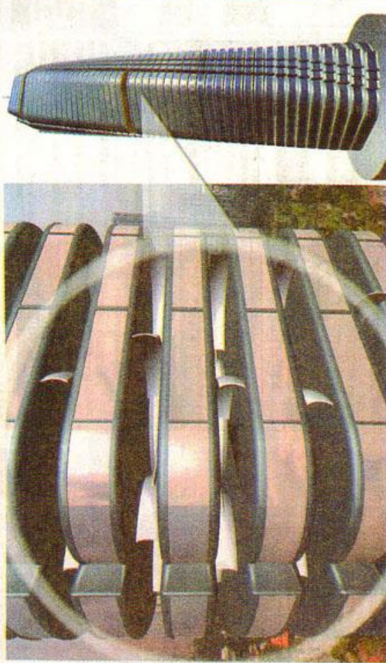
In a project to be unveiled today, Italian-Israeli architect David Fisher has dreamed up a 68-story hotel where each floor will rotate according to the preference of its occupants, causing the building's shape to constantly change.
