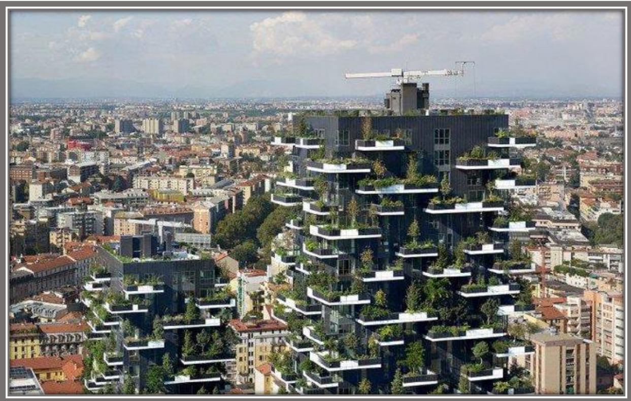
Figure 32:photo de premier foret vertical
