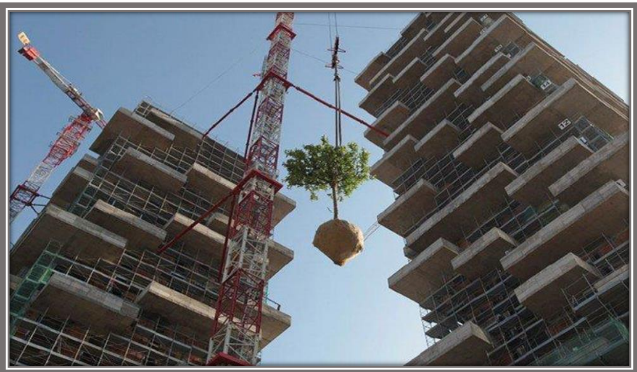
Figure 31:photo de premier foret vertical
