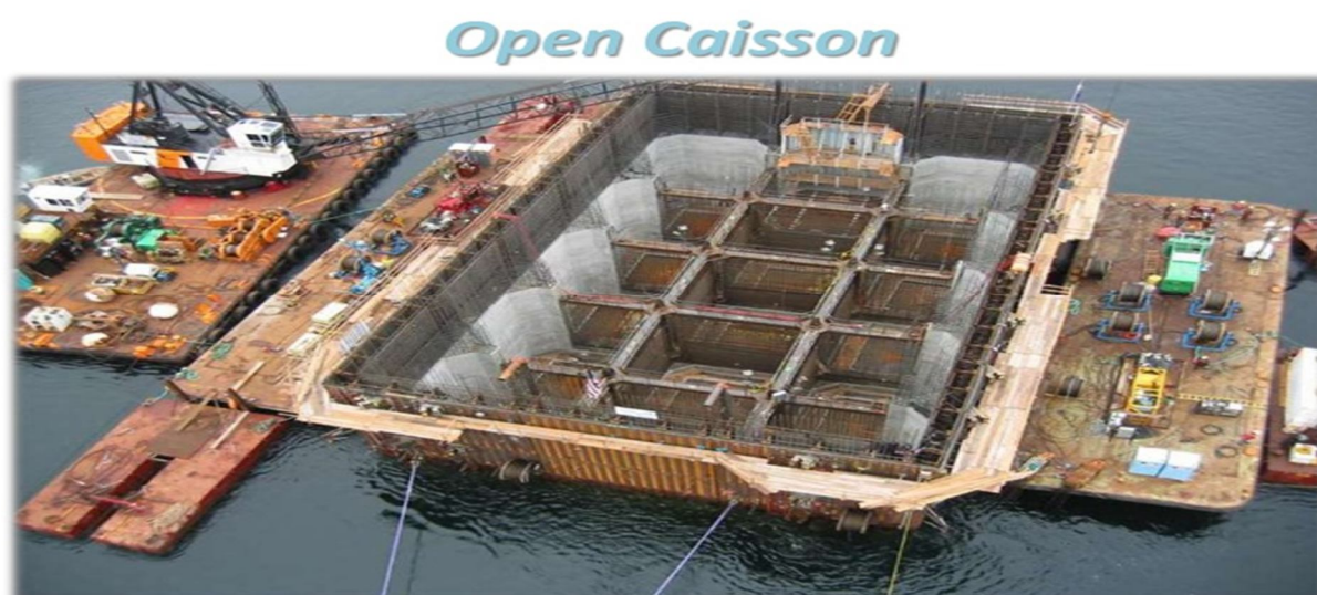
Figure 2.3 Caisson ouvert
