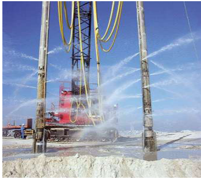
Figure I-26 La vibro-flottation (vibro-compaction)
