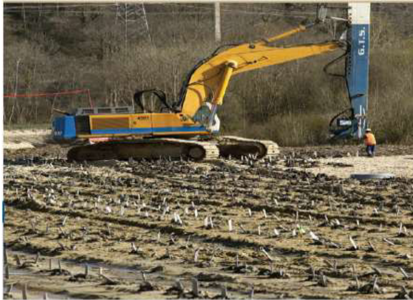
Figure I-31 drains verticaux
