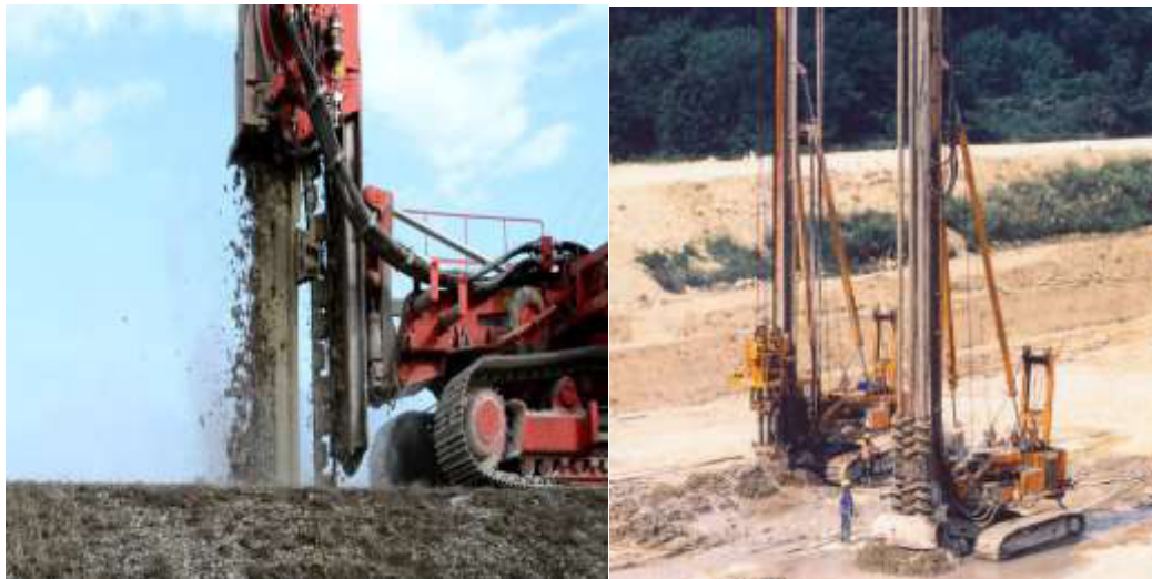
Figure I-28 Soil Mixing et Trench-mix
