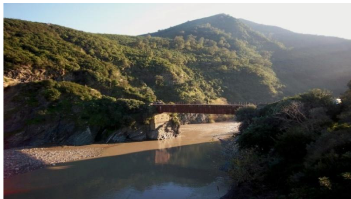
Figure 10: Photo du site (02)
