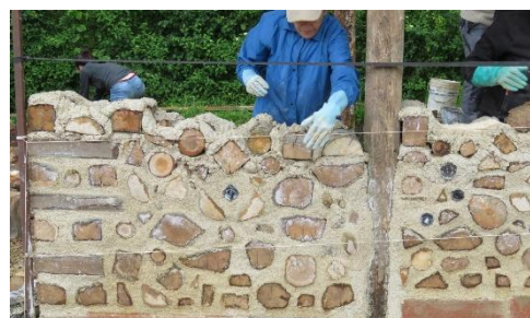
Figure 47: la technique du bois cordé / source : http://www.naturalbuildingblog.com/cordwood-barn
