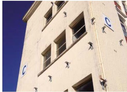
Figure 4.10: fixation des caissons.
