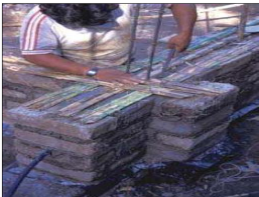
photo20 : Renforcement horizontal 38
