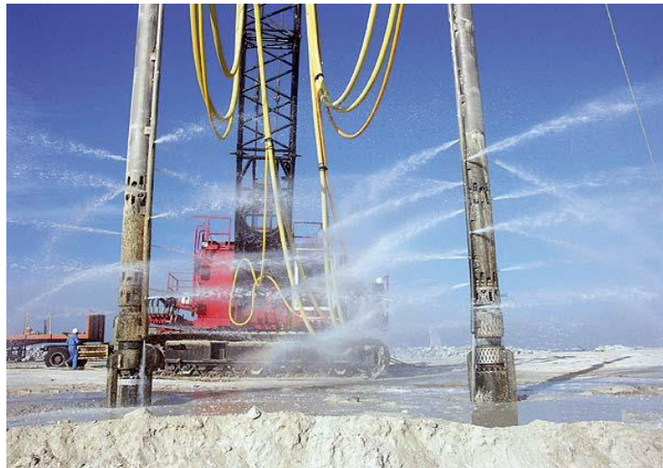
Figure I.35 La vibro-flottation (vibro-compaction)
