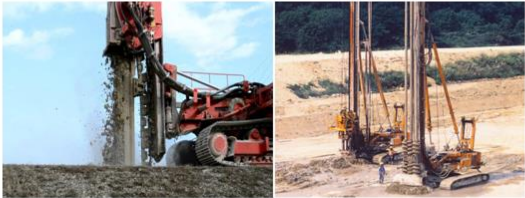
Figure I.37 Soil Mixing et Trench-mix
