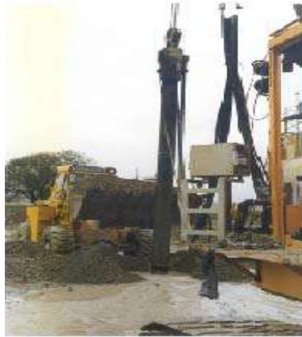
Figure I.8. Chantier de vibro-compaction.
