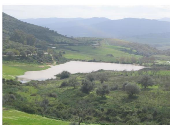
Figure 09 : La retenue collinaire de Sattara, Jijel (C.F.W, 2020).
