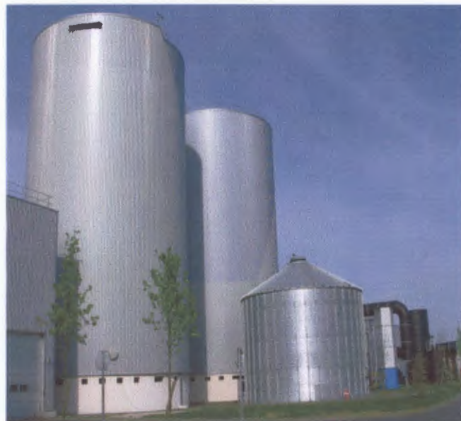
Figure 6: Digesteur vertical (site web 4)
